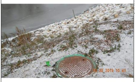
Inspect ID: MINR\_2019\_a\_0051 Title: USACE\_CEMVP\_MINR\_2019\_a\_0051\_1.jpg Rated Item: 3. Encroachments Caption: Rating: Unacceptable; Remarks: Sewer pipe in levee embankment; Action: Verify levee easement. Relocate encroachments/debris outside of levee easement; Station 1: 796+98
