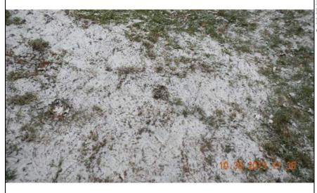
**Inspect ID:** MINR\_2019\_a\_0069 **Title:** USACE\_CEMVP\_MINR\_2019\_a\_0069\_1.jpg **Rated Item:** 10. Animal Control **Caption:** Rating: Minimally Acceptable; Remarks: Large animal burrow; Action: Excavate, inspect, backfill, compact in lifts, and reseed with grass; Improve animal burrow control program; Station\_1: 714+07
