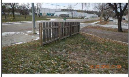
Inspect ID: MINR\_2019\_a\_0102 Title: USACE\_CEMVP\_MINR\_2019\_a\_0102\_7.jpg Rated Item: 3. Encroachments Caption: Rating: Unacceptable; Remarks: Multiple encroachment (light and power poles, fire hydrant, residential, fence and debris) along the levee alignment; Action: Verify levee easement. Relocate encroachments/debris outside of levee easement, unless approved by the Corps; Station 1: 625+70; Station 2: 643+37
