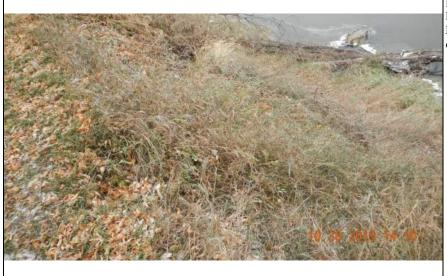
**Inspect ID:** MINR\_2019\_a\_0138 **Title:** USACE\_CEMVP\_MINR\_2019\_a\_0138\_1.jpg **Rated Item:** 6. Erosion/ Bank Caving **Caption:** Rating: Unacceptable; Remarks: Riverward slope eroded. Levee crown is less than 5 feet wide; Action: Preform an engineering evaluation of the areas and perform remedial action; Station 1: 545+00
