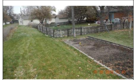
**Inspect ID:** MINR\_2019\_a\_0127 **Title:** USACE\_CEMVP\_MINR\_2019\_a\_0127\_1.jpg **Rated Item:** 2. Sod Cover **Caption:** Rating: Unacceptable; Remarks: Sod appears to have been deliberately removed to place a garden at the landside levee toe; Action: Reestablish sod cover
