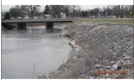
Inspect ID: MINR\_2019\_a\_0073 Title: USACE\_CEMVP\_MINR\_2019\_a\_0073\_1.jpg Rated Item: 6. Erosion/ Bank Caving Caption: Rating: Unacceptable; Remarks: Erosion along the levee crown and localized slope instability with steep sloughing riverside levee slope and channel bank; Action: Conduct an engineering evaluation of the erosion and slope stability. Complete remedial action to ensure a stable slope; Station\_1: 703+70
