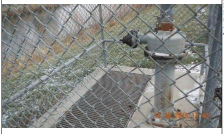
Inspect ID: MINR\_2019\_a\_0074 Title: USACE\_CEMVP\_MINR\_2019\_a\_0074\_1.jpg Rated Item: 13. Other Metallic Items Caption: Rating: Minimally Acceptable; Remarks: Gate well crank appears to be in good condition; however, gate well height indicator has been replaced by opaque metal pole, requiring operator to look into well; Action: Determine method of operation that does not require the operator to work over an open well (OSHA compliance); Station 1: 697+93
