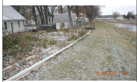
Inspect ID: MINR\_2019\_a\_0058 Title: USACE\_CEMVP\_MINR\_2019\_a\_0058\_3.jpg Rated Item: 3. Encroachments Caption: Rating: Unacceptable; Remarks: Fences, residential debris, power poles, flower beds, irrigation lines, and houses next to and/or on top of levee. Emergency operations will be impeded by these encroachments; Action: Verify location levee easement. Remove or relocate encroachments outside of the levee easement; Station 1: 761+00; Station 2: 770+50
