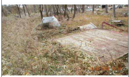
**Inspect ID:** MINR\_2019\_a\_0140 **Title:** USACE\_CEMVP\_MINR\_2019\_a\_0140\_1.jpg **Rated Item:** 3. Encroachments **Caption:** Rating: Minimally Acceptable; Remarks: Materials and debris placed along the toe of the levee; Action: Verify levee easement. Relocate encroachments/debris outside of levee easement; Station 1: 541+00
