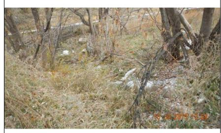
Inspect ID: MINR\_2019\_a\_0134 Title: USACE\_CEMVP\_MINR\_2019\_a\_0134\_2.jpg Rated Item: 3. Encroachments Caption: Rating: Unacceptable; Remarks: Portion of levee removed for interior drainage. NOTE: Construction activities and multiple lines of exposed pipe laid in dug drainage channel; Action: Verify levee easement. Replace portion of levee that has been removed; Station\_1: 545+00
