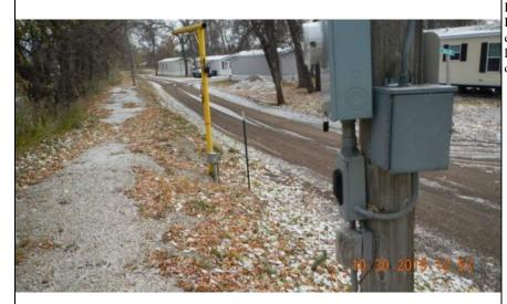
**Inspect ID:** MINR\_2019\_a\_0102 **Title:** USACE\_CEMVP\_MINR\_2019\_a\_0102\_2.jpg **Rated Item:** 3. Encroachments **Caption:** Rating: Unacceptable; Remarks: Multiple encroachment (light and power poles, fire hydrant, residential, fence and debris) along the levee alignment; Action: Verify levee easement. Relocate encroachments/debris outside of levee easement, unless approved by the Corps; Station 1: 625+70; Station 2: 643+37
