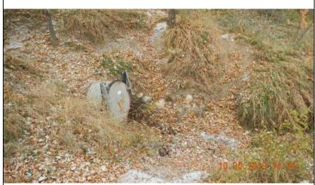
**Inspect ID:** MINR\_2019\_a\_0137 **Title:** USACE\_CEMVP\_MINR\_2019\_a\_0137\_1.jpg **Rated Item:** 6. Erosion/ Bank Caving **Caption:** Rating: Unacceptable; Remarks: Significant erosion has occured in levee slope around culvert; Action: Restore levee section. Install appropriate energy dissipation method with Corps approval if culvert is on plans; Station\_1: 563+00
