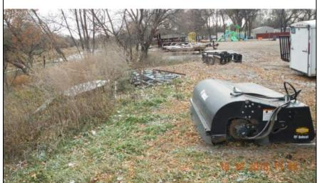
Inspect ID: MINR\_2019\_a\_0133 Title: USACE\_CEMVP\_MINR\_2019\_a\_0133\_1.jpg Rated Item: 3. Encroachments Caption: Rating: Unacceptable; Remarks: White fence added in 2016 at levee toe and construction materials have not been removed.; Action: Verify levee easement. Relocate encroachments/debris outside of levee easement; Station 1: 565+43
