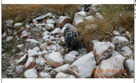
Inspect ID: MINR\_2019\_a\_0090 Title: USACE\_CEMVP\_MINR\_2019\_a\_0090\_1.jpg Rated Item: 3. Encroachments Caption: Rating: Minimally Acceptable; Remarks: PVC pipe through levee at toe. Flap gate placed on pipe in 2019; Action: Verify levee easement; Relocate encroachments outside of levee easement unless approved by Corps; Station 1: 676+91
