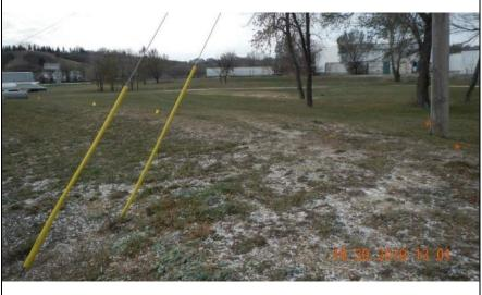
Inspect ID: MINR\_2019\_a\_0102 Title: USACE\_CEMVP\_MINR\_2019\_a\_0102\_9.jpg Rated Item: 3. Encroachments Caption: Rating: Unacceptable; Remarks: Multiple encroachment (light and power poles, fire hydrant, residential, fence and debris) along the levee alignment; Action: Verify levee easement. Relocate encroachments/debris outside of levee easement, unless approved by the Corps; Station 1: 625+70; Station 2: 643+37
