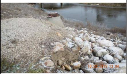
**Inspect ID:** MINR\_2019\_a\_0110 **Title:** USACE\_CEMVP\_MINR\_2019\_a\_0110\_1.jpg **Rated Item:** 3. Encroachments **Caption:** Rating: Unacceptable; Remarks: Manhole has been placed in levee slope; Action: Verify levee easement. Relocate encroachment outside of levee easement, unless approved by the Corps; Station 1: 624+00
