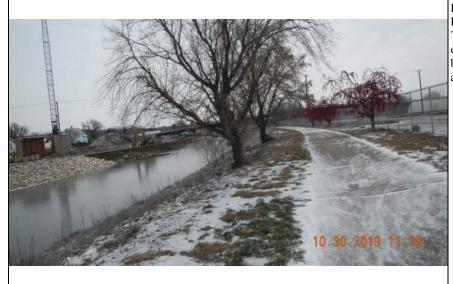
Inspect ID: MINR\_2019\_a\_0066 Title: USACE\_CEMVP\_MINR\_2019\_a\_0066\_2.jpg Rated Item: 1. Unwanted Vegetation Growth Caption: Rating: Unacceptable; Remarks: Trees along the top of the channel bank within the easement area; Action: Verify channel easement; Remove unwanted vegetation up to the channe easement. Remove root ball, backfill, compact in lifts, and reseed with grass. Ensure environmental compliance with all appropriate agencies prior to removal; Station 1:717+00; Station 2:740+00
