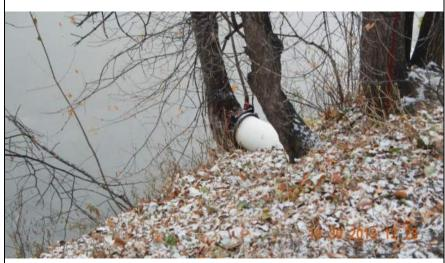
Inspect ID: MINR\_2019\_a\_0092 Title: USACE\_CEMVP\_MINR\_2019\_a\_0092\_1.jpg Rated Item: 3. Encroachments Caption: Rating: Minimally Acceptable; Remarks: PVC pipe through levee embankment. Flap gate placed on end of the pipe in 2019; Action: Verify levee easement. Determine origin of the pipe and relocate encroachments outside of easement unless approved by Corps; Station 1: 670+00
