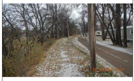
Inspect ID: MINR\_2019\_a\_0102 Title: USACE\_CEMVP\_MINR\_2019\_a\_0102\_1.jpg Rated Item: 3. Encroachments Caption: Rating: Unacceptable; Remarks: Multiple encroachment (light and power poles, fire hydrant, residential, fence and debris) along the levee alignment; Action: Verify levee easement. Relocate encroachments/debris outside of levee easement, unless approved by the Corps; Station 1: 625+70; Station 2: 643+37
