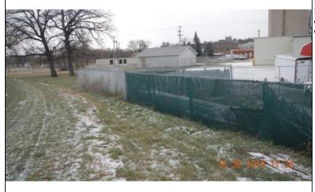
Inspect ID: MINR\_2019\_a\_0149 Title: USACE\_CEMVP\_MINR\_2019\_a\_0149\_1.jpg Rated Item: 3. Encroachments Caption: Rating: Unacceptable; Remarks: Fence and debris at landside levee toe; Action: Verify levee easement; Relocate encroachments outside of levee easement; Station 1: 714+07; Station 2: 715+48
