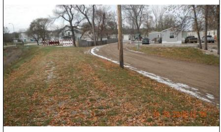
**Inspect ID:** MINR\_2019\_a\_0102 **Title:** USACE\_CEMVP\_MINR\_2019\_a\_0102\_5.jpg **Rated Item:** 3. Encroachments **Caption:** Rating: Unacceptable; Remarks: Multiple encroachment (light and power poles, fire hydrant, residential, fence and debris) along the levee alignment; Action: Verify levee easement. Relocate encroachments/debris outside of levee easement, unless approved by the Corps; Station 1: 625+70; Station 2: 643+37
