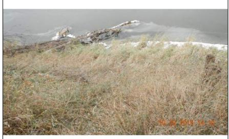
**Inspect ID:** MINR\_2019\_a\_0138 **Title:** USACE\_CEMVP\_MINR\_2019\_a\_0138\_2.jpg **Rated Item:** 6. Erosion/ Bank Caving **Caption:** Rating: Unacceptable; Remarks: Riverward slope eroded. Levee crown is less than 5 feet wide; Action: Preform an engineering evaluation of the areas and perform remedial action; Station\_1: 545+00
