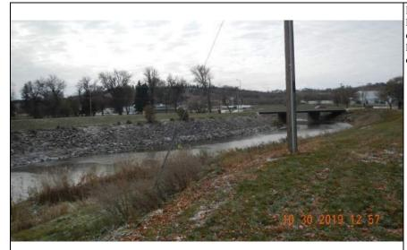
Inspect ID: MINR\_2019\_a\_0102 Title: USACE\_CEMVP\_MINR\_2019\_a\_0102\_4.jpg Rated Item: 3. Encroachments Caption: Rating: Unacceptable; Remarks: Multiple encroachment (light and power poles, fire hydrant, residential, fence and debris) along the levee alignment; Action: Verify levee easement. Relocate encroachments/debris outside of levee easement, unless approved by the Corps; Station 1: 625+70; Station 2: 643+37
