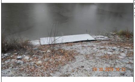
Inspect ID: MINR\_2019\_a\_0040 Title: USACE\_CEMVP\_MINR\_2019\_a\_0040\_1.jpg Rated Item: 3. Encroachments Caption: Rating: Unacceptable; Remarks: Boat dock driven into riverside levee slope. Steps and other residential debris on slope as well; Action: Verify levee easement. Relocate encroachments/debris outside of levee easement; Station 1: 819+61
