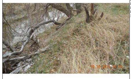
Inspect ID: MINR\_2019\_a\_0141 Title: USACE\_CEMVP\_MINR\_2019\_a\_0141\_1.jpg Rated Item: 6. Erosion/Bank Caving Caption: Rating: Unacceptable; Remarks: Erosion of the levee riverside toe and slope; levee crest less than 3 foot wide; Action: Preform an engineering evaluation of the areas and perform remedial action; Station\_1: 541+00
