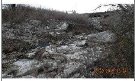
**Inspect ID:** MINR\_2019\_a\_0115 **Title:** USACE\_CEMVP\_MINR\_2019\_a\_0115\_2.jpg **Rated Item:** 2. Shoaling (sediment deposition) **Caption:** Rating: Unacceptable; Remarks: Bank erosion is causing shoaling within the channel that is diverting flow towards the left bank, resulting in left bank erosion; Action: Remove shoaling. Restore channel to the design grade and cross section. Ensure environmental compliance with all appropriate agencies prior to removal; Station 1: 601+35
