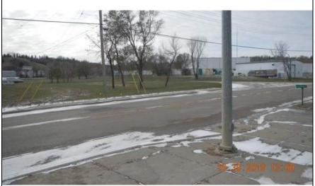
Inspect ID: MINR\_2019\_a\_0102 Title: USACE\_CEMVP\_MINR\_2019\_a\_0102\_6.jpg Rated Item: 3. Encroachments Caption: Rating: Unacceptable; Remarks: Multiple encroachment (light and power poles, fire hydrant, residential, fence and debris) along the levee alignment; Action: Verify levee easement. Relocate encroachments/debris outside of levee easement, unless approved by the Corps; Station\_1: 625+70; Station\_2: 643+37
