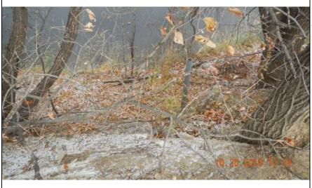
**Inspect ID:** MINR\_2019\_a\_0152 **Title:** USACE\_CEMVP\_MINR\_2019\_a\_0152\_2.jpg **Rated Item:** 6. Erosion/Bank Caving **Caption:** Rating: Unacceptable; Remarks: Erosion and steep channel bank along the riverside levee slope; Action: Evaluate steep bank and flatten slope. Backfill erosion to design grade, compact in lifts, and evaluate the need for erosion protection; Station 1: 633+96; Station 2: 643+69
