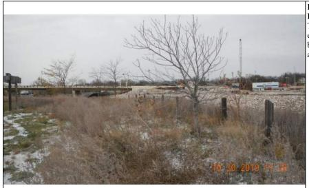
Inspect ID: MINR\_2019\_a\_0066 Title: USACE\_CEMVP\_MINR\_2019\_a\_0066\_1.jpg Rated Item: 1. Unwanted Vegetation Growth Caption: Rating: Unacceptable; Remarks: Trees along the top of the channel bank within the easement area; Action: Verify channel easement; Remove unwanted vegetation up to the channe easement. Remove root ball, backfill, compact in lifts, and reseed with grass. Ensure environmental compliance with all appropriate agencies prior to removal; Station 1: 717+00; Station 2: 740+00
