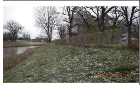
Inspect ID: MINR\_2019\_a\_0058 Title: USACE\_CEMVP\_MINR\_2019\_a\_0058\_1.jpg Rated Item: 3. Encroachments Caption: Rating: Unacceptable; Remarks: Fences, residential debris, power poles, flower beds, irrigation lines, and houses next to and/or on top of levee. Emergency operations will be impeded by these encroachments; Action: Verify location levee easement. Remove or relocate encroachments outside of the levee easement; Station\_1: 761+00; Station\_2: 770+50
