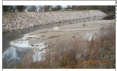
Inspect ID: MINR\_2019\_a\_0115 Title: USACE\_CEMVP\_MINR\_2019\_a\_0115\_1.jpg Rated Item: 2. Shoaling (sediment deposition) Caption: Rating: Unacceptable; Remarks: Bank erosion is causing shoaling within the channel that is diverting flow towards the left bank, resulting in left bank erosion; Action: Remove shoaling. Restore channel to the design grade and cross section. Ensure environmental compliance with all appropriate agencies prior to removal; Station 1: 601+35
