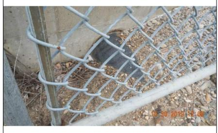
Inspect ID: MINR\_2019\_a\_0084 Title: USACE\_CEMVP\_MINR\_2019\_a\_0084\_1.jpg Rated Item: 6. Erosion/ Bank Caving Caption: Rating: Unacceptable; Remarks: Erosion and bank caving along the levee toe. Force main exposed due to erosion at pump station gate; Action: Backfill erosion to the design grade, compact in lifts, and re-sod; Reevaluate drainage and erosion protection; Station 1: Little Rosevelt PS
