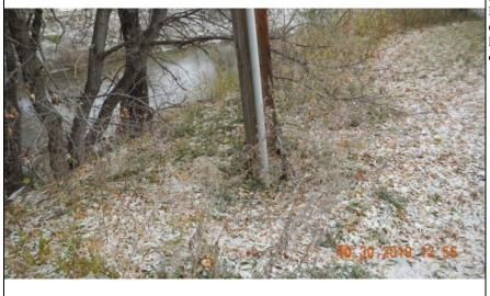
**Inspect ID:** MINR\_2019\_a\_0102 **Title:** USACE\_CEMVP\_MINR\_2019\_a\_0102\_3.jpg **Rated Item:** 3. Encroachments **Caption:** Rating: Unacceptable; Remarks: Multiple encroachment (light and power poles, fire hydrant, residential, fence and debris) along the levee alignment; Action: Verify levee easement. Relocate encroachments/debris outside of levee easement, unless approved by the Corps; Station 1: 625+70; Station 2: 643+37
