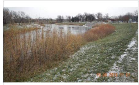
**Inspect ID:** MINR\_2019\_a\_0077 **Title:** USACE\_CEMVP\_MINR\_2019\_a\_0077\_1.jpg **Rated Item:** 1. Unwanted Vegetation Growth **Caption:** Rating: Minimally Acceptable; Remarks: Overgrown vegetation growing at riverside toe of levee prevents inspection to water's edge; Action: Mow grass on a routine basis and maintain in compliance with operation and maintenance manual (A=0-6", M=6"-12",
