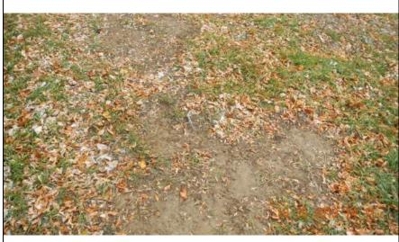
**Inspect ID:** MINR 2019 a 0139 **Title:** USACE\_CEMVP\_MINR 2019 a 0139 1.jpg **Rated Item:** 8. Depressions/ Rutting **Caption:** Rating: Minimally Acceptable; Remarks: Depression and rutting on levee crown,; Action: Backfill ruts/depression to the design grade, compact in lifts, and re-sod; Reevaluate levee crown surface; A resilient surface treatment is recommended for levee activities; Station 1: 560+00
