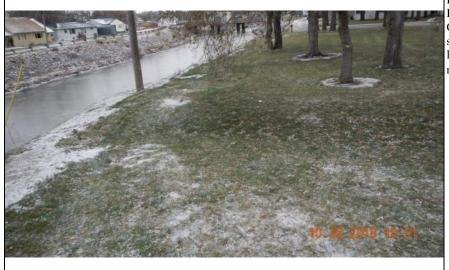
Inspect ID: MINR\_2019\_a\_0054 Title: USACE\_CEMVP\_MINR\_2019\_a\_0054\_1.jpg Rated Item: 4. Closure Structures (Stop Log, Earthen Closures, Gates, or Sandbag Closures) (A or U only) Caption: Rating: Unacceptable; Remarks: Discontinuous levee section. A closure would be required to utilize protection offered by the discontinuous levee section; Action: Evaluate the level of protection and determine when closures need to be installed; Station 1: 784+15
