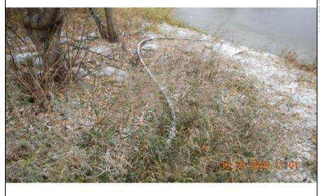
**Inspect ID:** MINR\_2019\_a\_0057 **Title:** USACE\_CEMVP\_MINR\_2019\_a\_0057\_1.jpg **Rated Item:** 3. Encroachments **Caption:** Rating: Minimally Acceptable; Remarks: Irrigation line on top of levee; Action: Monitor irrigation line and prevent homeowner from trenching into the levee or eroding out the levee embankment; Station 1: 770+55
