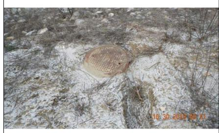
Inspect ID: MINR\_2019\_a\_0014 Title: USACE\_CEMVP\_MINR\_2019\_a\_0014\_1.jpg Rated Item: 3. Encroachments Caption: Rating: Unacceptable; Remarks: Sewer manhole located at levee crown. Sponsor indicated this portion of levee will be abandoned with new design; Action: Verify levee easement. Relocate encroachments/debris outside of levee easement. Verify approval was received from Corps to perform excavations; Station\_1: 847+38
