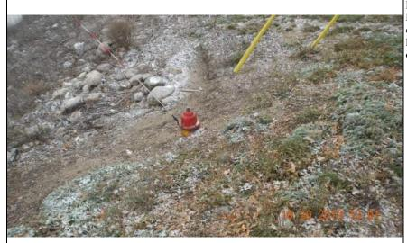
**Inspect ID:** MINR\_2019\_a\_0102 **Title:** USACE\_CEMVP\_MINR\_2019\_a\_0102\_8.jpg **Rated Item:** 3. Encroachments **Caption:** Rating: Unacceptable; Remarks: Multiple encroachment (light and power poles, fire hydrant, residential, fence and debris) along the levee alignment; Action: Verify levee easement. Relocate encroachments/debris outside of levee easement, unless approved by the Corps; Station 1: 625+70; Station 2: 643+37
