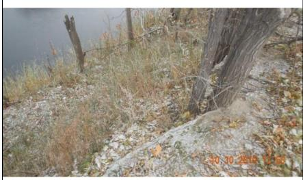
**Inspect ID:** MINR\_2019\_a\_0152 **Title:** USACE\_CEMVP\_MINR\_2019\_a\_0152\_1.jpg **Rated Item:** 6. Erosion/Bank Caving **Caption:** Rating: Unacceptable; Remarks: Erosion and steep channel bank along the riverside levee slope; Action: Evaluate steep bank and flatten slope. Backfill erosion to design grade, compact in lifts, and evaluate the need for erosion protection; Station 1: 633+96; Station 2: 643+69
