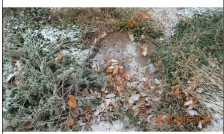
**Inspect ID:** MINR\_2019\_a\_0050 **Title:** USACE\_CEMVP\_MINR\_2019\_a\_0050\_1.jpg **Rated Item:** 3. Encroachments **Caption:** Rating: Unacceptable; Remarks: Sewer manhole in levee crown; Action: Verify levee easement. Relocate encroachments/debris outside of levee easement; Station 1: 798+15
