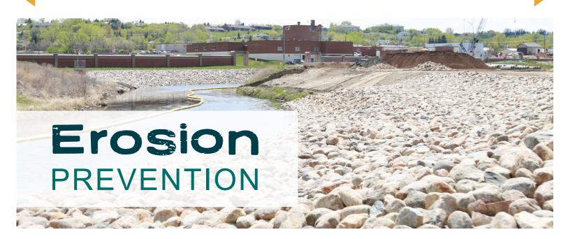
A layer of stones, also known as riprap, is many times installed along riverbanks or lake shores to prevent erosion. The larger the stones the more resistant the stones are to movement and therefore can protect a riverbank from flood events or a lake shore from waves.
