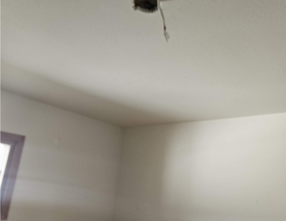
Photo 5. Ceiling drywall example.
