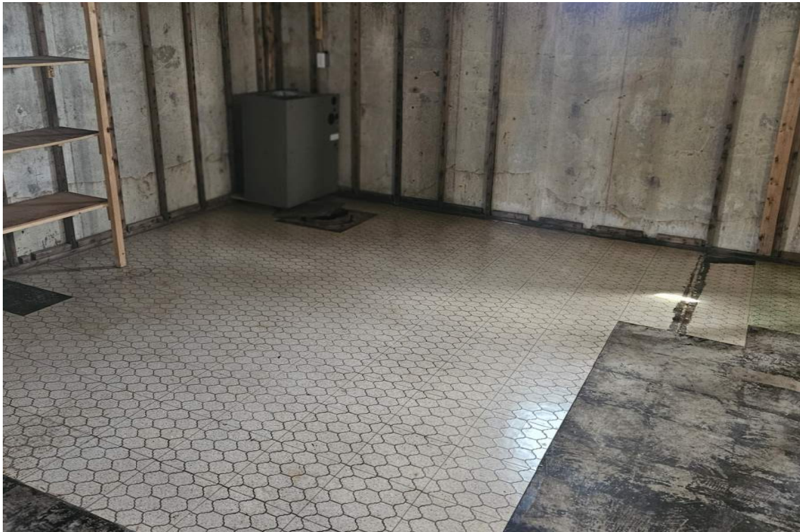
Photo 4 12" x 12" VCT tiles in basement.
