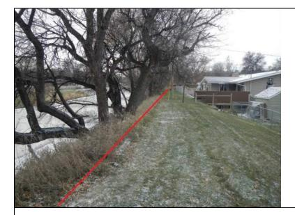
Inspect ID: MINL\_2019\_a\_0101 Title: USACE\_CEMVP\_MINL\_2019\_a\_0101\_1.jpg Rated Item: 1. Unwanted Vegetation Growth Caption: Rating: Unacceptable; Remarks: Large trees located on the riverside slope of the levee embankment; Action: Remove large tree from vegetation-free zone, up to the levee easement. Remove root ball, backfill, compact in lifts, and reseed with grass. Ensure environmental compliance with all appropriate agencies prior to removal; Station\_1: 791+07L; Station\_2: 794+21L
