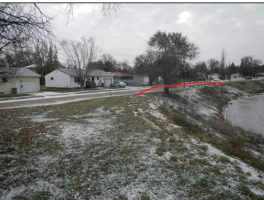
Inspect ID: MINL\_2019\_a\_0127 Title: USACE\_CEMVP\_MINL\_2019\_a\_0127\_1.jpg Rated Item: 4. Closure Structures (Stop Log, Earthen Closures, Gates, or Sandbag Closures) (A or U only) Caption: Rating: Unacceptable; Remarks: Discontinuous levee section. A closure would be required to utilize protection offered by the discontinuous levee section; Action: Evaluate the level of protection and determined when closures need to be installed; Station 1: 620+24L; Station 2: 624+24L
