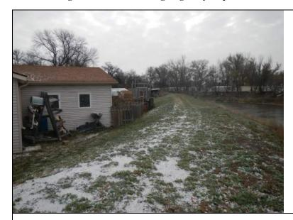
Inspect ID: MINL\_2019\_a\_0124 Title: USACE\_CEMVP\_MINL\_2019\_a\_0124\_1.jpg Rated Item: 3. Encroachments Caption: Rating: Unacceptable; Remarks: Multiple encroachments along the levee side toe; Action: Verify levee easement. Relocate encroachment structures outside of levee easement, unless approved by Corps; Station\_1: 643+92L; Station 2: 647+52L
