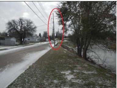
Inspect ID: MINL\_2019\_a\_0079 Title: USACE\_CEMVP\_MINL\_2019\_a\_0079\_1.jpg Rated Item: 3. Encroachments Caption: Rating: Unacceptable; Remarks: Power poles and guard rail on levee crown; Action: Verify levee easement; Relocate encroachments outside of levee easement, unless approved by Corps; Station 1: 633+41L
