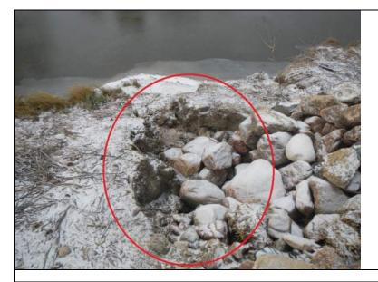
Inspect ID: MINL\_2019\_a\_0045 Title: USACE\_CEMVP\_MINL\_2019\_a\_0045\_1.jpg Rated Item: 6. Erosion/ Bank Caving Caption: Rating: Minimally Acceptable; Remarks: Erosion has occured at the end of interior drainage culvert; Action: Extend erosion protection down to water surface to prevent further loss of material; Station\_1: 711+83; ;;
