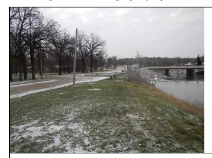
Inspect ID: MINL\_2019\_a\_0070 Title: USACE\_CEMVP\_MINL\_2019\_a\_0070\_1.jpg Rated Item: 3. Encroachments Caption: Rating: Unacceptable; Remarks: Power pole levee alignment; Action: Verify levee easement; Relocate encroachments/debris outside of levee easement, unless approved by Corps; Station 1: 648+32L
