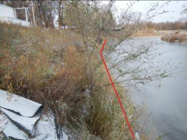
Inspect ID: MINL\_2019\_a\_0098 Title: USACE\_CEMVP\_MINL\_2019\_a\_0098\_1.jpg Rated Item: 6. Erosion/Bank Caving Caption: Rating: Unacceptable; Remarks: Erosion and bank caving along the left channel bank and levee riverside slope and toe; Action: Backfill erosion to the design grade, compact in lifts, and evaluate if riprap is needed or reseed; Station 1: 815+33L; Station 2: 818.06L
