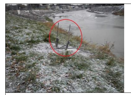
Inspect ID: MINL\_2019\_a\_0020 Title: USACE\_CEMVP\_MINL\_2019\_a\_0020\_1.jpg Rated Item: 3. Encroachments Caption: Rating: Unacceptable; Remarks: Irrigation pumps and lines through levee; Action: Verify levee easement; Relocate encroachments outside of levee easement; Station 1: 789+90L
