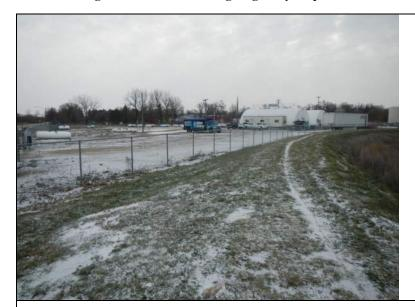
Inspect ID: MINL\_2019\_a\_0117 Title: USACE\_CEMVP\_MINL\_2019\_a\_0117\_1.jpg Rated Item: 3. Encroachments Caption: Rating: Unacceptable; Remarks: A fence is located at the landside toe of the levee embankment; Action: Verify levee easement. Relocate fence encroachment outside of levee easement, unless approved by Corps; Station 1: 676+63L; Station 2: 680+78L
