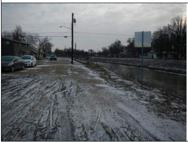
Inspect ID: MINL\_2019\_a\_0106 Title: USACE\_CEMVP\_MINL\_2019\_a\_0106\_1.jpg Rated Item: 4. Closure Structures (Stop Log, Earthen Closures, Gates, or Sandbag Closures) (A or U only) Caption: Rating: Unacceptable; Remarks: Discontinuous levee section. A closure would be required to utilize protection offered by the discontinuous levee section; Action: Evaluate the level of protection and determine when closures need to be installed; Station 1: 773+39L; Station 2: 784+37L
