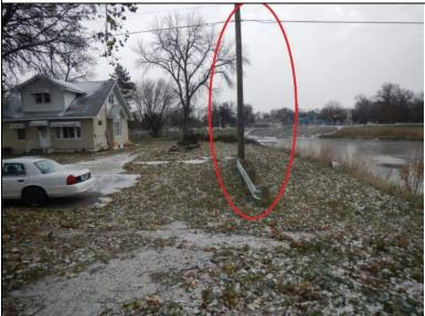
**Inspect ID:** MINL 2019 a 0052 **Title:** USACE CEMVP MINL 2019 a 0052 1.jpg **Rated Item:** 3. Encroachments **Caption:** Rating: Unacceptable; Remarks: Guard rail and power pole on levee; Action: Verify levee easement; Relocate encroachments outside of levee easement; Station 1: 697+50
