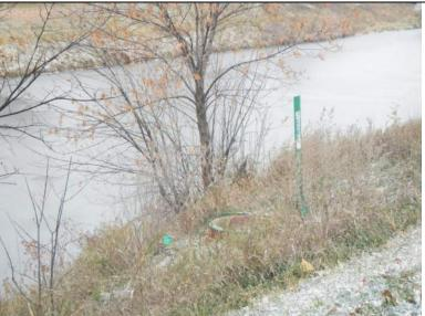
**Inspect ID:** MINL\_2019\_a\_0061 **Title:** USACE\_CEMVP\_MINL\_2019\_a\_0061\_1.jpg **Rated Item:** 3. Encroachments **Caption:** Rating: Unacceptable; Remarks: Sewer manhole on riverside levee slope; Action: Verify levee easement; Relocate encroachments outside of levee easement; Station 1: 675+42L
