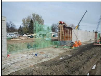
Inspect ID: MINL 2019 a 0110 Title: USACE\_CEMVP\_MINL 2019 a 0110 2.jpg Rated Item: 3. Encroachments Caption: Rating: Acceptable; Remarks: Area under construction for new levee and pump station construction. Approved as part of the 408 modification to the existing project; Action: Construct project per the approved plans and specifications; Station 1: 717+33L; Station 2: 759+15L
