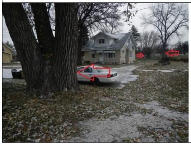
Inspect ID: MINL\_2019\_a\_0051 Title: USACE\_CEMVP\_MINL\_2019\_a\_0051\_1.jpg Rated Item: 1. Unwanted Vegetation Growth Caption: Rating: Unacceptable; Remarks: Large tree within the vegetation-free zone; Action: Remove large tree from vegetation-free zone, up to the levee easement. Remove root ball, backfill, compact in lifts, and reseed with grass. Ensure environmental compliance with all appropriate agencies prior to removal; Station 1: 697+50
