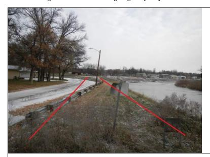
Inspect ID: MINL\_2019\_a\_0103 Title: USACE\_CEMVP\_MINL\_2019\_a\_0103\_1.jpg Rated Item: 4. Closure Structures (Stop Log, Earthen Closures, Gates, or Sandbag Closures) (A or U only) Caption: Rating: Unacceptable; Remarks: Discontinuous levee section. A closure would be required to utilize protection offered by the discontinuous levee section; Action: Evaluate the level of protection and determine when closures need to be installed; Station 1: 789+36L; Station 2: 791+30L
