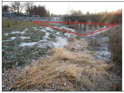
Inspect ID: MINL\_2019\_a\_0001 Title: USACE\_CEMVP\_MINL\_2019\_a\_0001\_1.jpg Rated Item: 3. Encroachments Caption: Rating: Unacceptable; Remarks: A drainage ditch was cut through the levee prism; Action: Fill and compact the cut area with appropriate material to design elevation, and reseed with grass; Station\_1: 828+60
