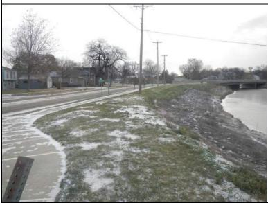
Inspect ID: MINL\_2019\_a\_0030 Title: USACE\_CEMVP\_MINL\_2019\_a\_0030\_1.jpg Rated Item: 3. Encroachments Caption: Rating: Unacceptable; Remarks: Power poles in levee crown; Action: Verify levee easement; Relocate encroachments/debris outside of levee easement, unless approved by Corps; Station 1: 777+31L
