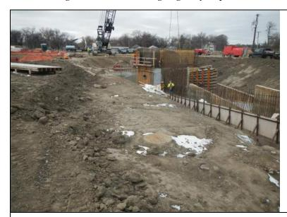
**Inspect ID:** MINL\_2019\_a\_0110 **Title:** USACE\_CEMVP\_MINL\_2019\_a\_0110\_1.jpg **Rated Item:** 3. Encroachments **Caption:** Rating: Acceptable; Remarks: Area under construction for new levee and pump station construction. Approved as part of the 408 modification to the existing project; Action: Construct project per the approved plans and specifications; Station\_1: 717+33L; Station\_2: 759+15L
