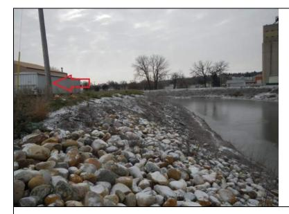
Inspect ID: MINL 2019 a 0044 Title: USACE CEMVP MINL 2019 a 0044 1.jpg Rated Item: 3. Encroachments Caption: Rating: Unacceptable; Remarks: Power pole on levee, Vegetation in riprap; Action: Verify levee easement, relocate encroachments outside of levee easement, unless approved by Corps,Remove unwanted vegetation from vegetation-free zone, Ensure environmental compliance with all appropriate agencies prior to removal; Station 1: 714+18
