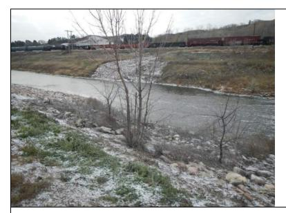
Inspect ID: MINL\_2019\_a\_0086 Title: USACE\_CEMVP\_MINL\_2019\_a\_0086\_1.jpg Rated Item: 1. Unwanted Vegetation Growth Caption: Rating: Unacceptable; Remarks: Large trees growing within the riverside levee slope; Action: Remove large trees from vegetation-free zone, up to the levee easement. Remove root ball and backfill with riprap. Ensure environmental compliance with
