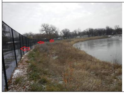
Inspect ID: MINL\_2019\_a\_0121 Title: USACE\_CEMVP\_MINL\_2019\_a\_0121\_1.jpg Rated Item: 3. Encroachments Caption: Rating: Acceptable; Remarks: Zoo fence located on top of the levee embankment. The fence has been approved by the Corps; Action: NA; Station 1: 09+81L; Station 2: 02+96L
