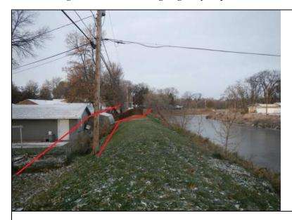
Inspect ID: MINL\_2019\_a\_0097 Title: USACE\_CEMVP\_MINL\_2019\_a\_0097\_1.jpg Rated Item: 3. Encroachments Caption: Rating: Unacceptable; Remarks: Residential encroachments, utility poles, fences, irregation lines, etc. along the entire levee reach; Action: Verify levee easement. Relocate encroachments outside of levee easement, unless approved by the Corps; Station 1: 813+77L; Station 2: 828+60L
