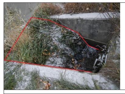
Inspect ID: MINL\_2019\_a\_0007 Title: USACE\_CEMVP\_MINL\_2019\_a\_0007\_1.jpg Rated Item: 1. Vegetation and Obstructions Caption: Rating: Minimally Acceptable; Remarks: Sediment and vegetation growth in discharge basin; Action: Remove vegetation and sedimentation from the drainage feature; Station 1: 818+85L
