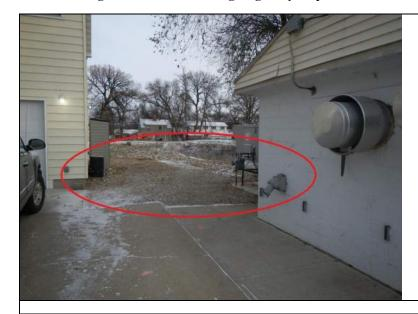
Inspect ID: MINL\_2019\_a\_0004 Title: USACE\_CEMVP\_MINL\_2019\_a\_0004\_1.jpg Rated Item: 3. Encroachments Caption: Rating: Unacceptable; Remarks: Low spot in levee crown and new garage next to levee; Action: Verify levee easement; Relocate encroachments/debris outside of levee easement, unless approved by Corps; Raise levee to design grade, compact in lifts, and reseed with grass; Station 1: 822+82L
