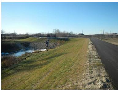
Inspect ID: MINL\_2019\_a\_0132 Title: USACE\_CEMVP\_MINL\_2019\_a\_0132\_1.jpg Rated Item: 3. Encroachments Caption: Rating: Acceptable; Remarks: Area under construction for new levee and pump station construction.approved as part of the 408 modification to the existing project; Action: Construct project per the approved plans and specifications; Station 1: 62+18L; Station 2: 829+03L
