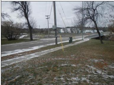
Inspect ID: MINL\_2019\_a\_0128 Title: USACE\_CEMVP\_MINL\_2019\_a\_0128\_1.jpg Rated Item: 3. Encroachments Caption: Rating: Unacceptable; Remarks: Power pole and utility box located within the alignment of levee; Action: Verify levee easement; Relocate encroachments/debris outside of levee easement, unless approved by Corps; Station 1: 625+42; ;;;;
