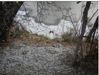
**Inspect ID:** MINL\_2019\_a\_0019 **Title:** USACE\_CEMVP\_MINL\_2019\_a\_0019\_1.jpg **Rated Item:** 3. Encroachments **Caption:** Rating: Unacceptable; Remarks: Interior drainage pipe through the levee embankment. Not
