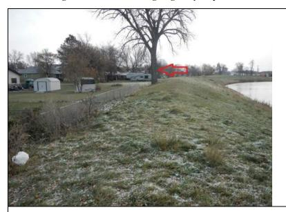
Inspect ID: MINL\_2019\_a\_0034 Title: USACE\_CEMVP\_MINL\_2019\_a\_0034\_1.jpg Rated Item: 1. Unwanted Vegetation Growth Caption: Rating: Unacceptable; Remarks: Large tree on the levee landside slope; Action: Remove large tree from vegetation-free zone, up to the levee easement. Remove root ball, backfill, compact in lifts, and reseed with grass. Ensure environmental compliance with all appropriate agencies prior to removal; Station 1: 765+00; ;;;;
