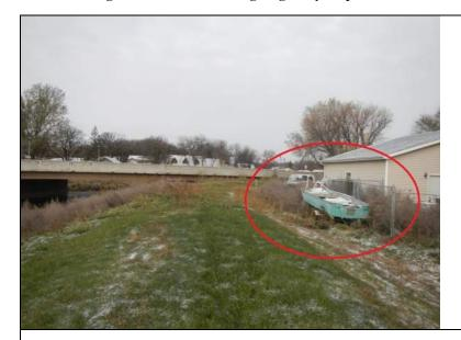
Inspect ID: MINL 2019 a 0107 Title: USACE CEMVP MINL 2019 a 0107 1.jpg Rated Item: 3. Encroachments Caption: Rating: Unacceptable; Remarks: Residential encroachments, structures, vehicles, power poles, and landscaping along the levee embankment; Action: Verify levee easement. Relocate encroachments outside of levee embankment, unless approved by the Corps; Station 1: 766+75L; Station 2: 773+23L
