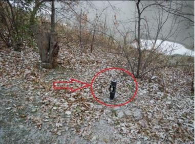
Inspect ID: MINL 2019 a 0009 Title: USACE CEMVP MINL 2019 a 0009 1.jpg Rated Item: 3. Encroachments Caption: Rating: Unacceptable; Remarks: Sump pump hose through levee; Action: Verify levee easement; Relocate encroachments/debris outside of levee easement, unless approved by Corps; Station 1: 815+33L
