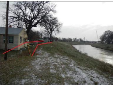
Inspect ID: MINL 2019 a 0107 Title: USACE CEMVP MINL 2019 a 0107 2.jpg Rated Item: 3. Encroachments Caption: Rating: Unacceptable; Remarks: Residential encroachments, structures, vehicles, power poles, and landscaping along the levee embankment; Action: Verify levee easement. Relocate encroachments outside of levee embankment, unless approved by the Corps; Station 1: 766+75L; Station 2: 773+23L
