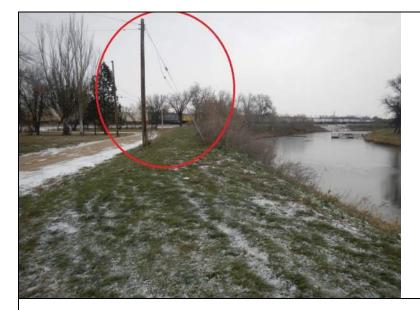
Inspect ID: MINL\_2019\_a\_0056 Title: USACE\_CEMVP\_MINL\_2019\_a\_0056\_1.jpg Rated Item: 3. Encroachments Caption: Rating: Unacceptable; Remarks: A utility pole is located in the levee prism; Action: Verify levee easement. Relocate utility pole outside of levee easement, unless approved by Corps; Station\_1: 686+53
