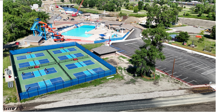
➤ View of new restroom and parking lot with entrances next to MCE tracks
