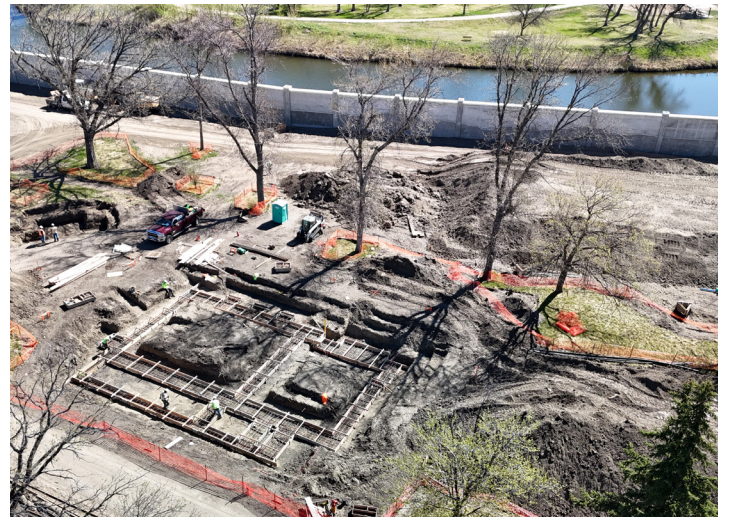
➤ North American cats exhibit footings being laid out
