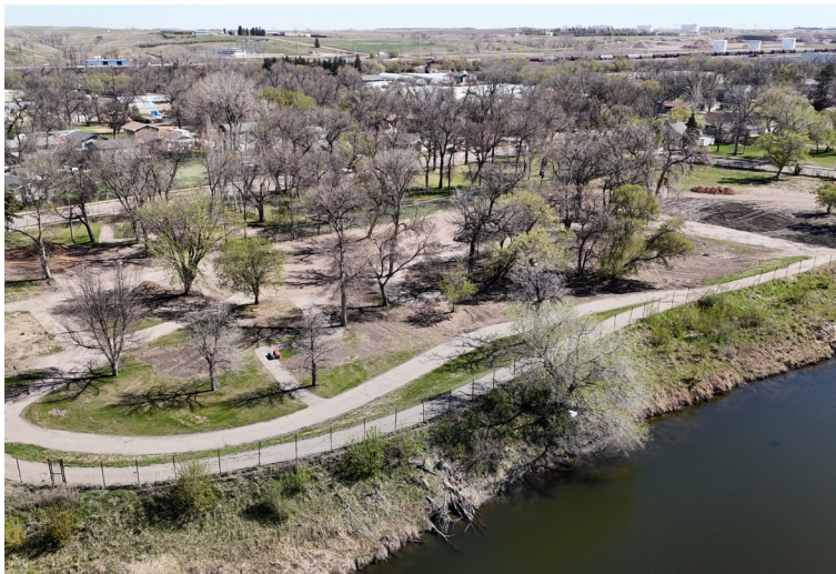
➤ Completed demolition of former North American exhibits
