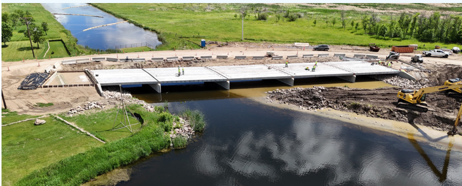
▼ Mouse River Park Bridge Construction July 2026
