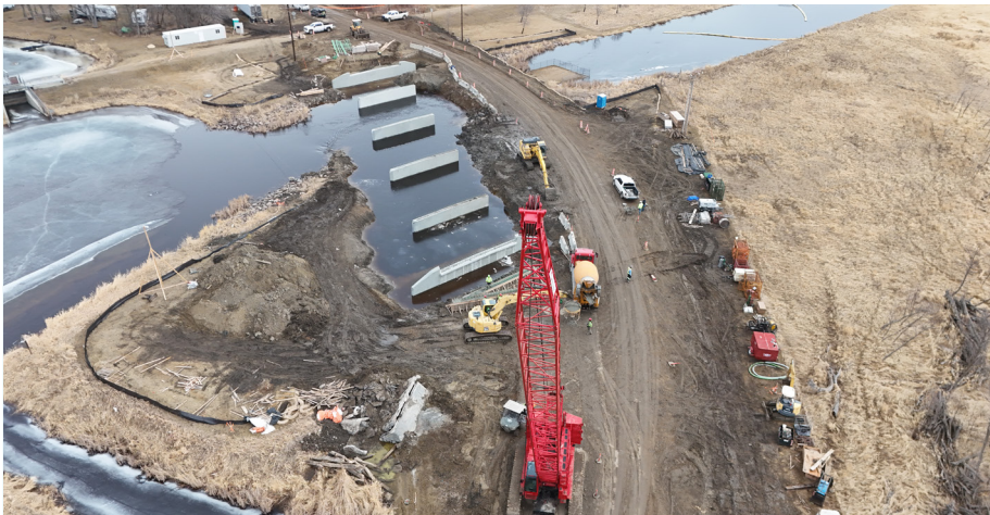
▲ Mouse River Park Bridge Construction March 2026
