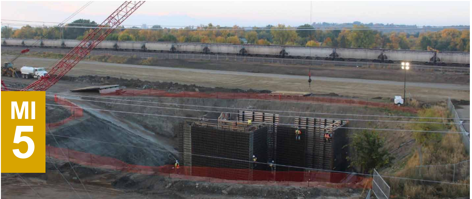
Storm water pump station under construction.
