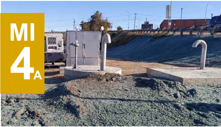
Sanitary Lift Station under construction.
