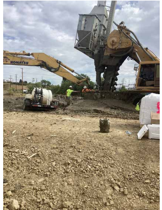
Impervious subsurface slurry seepage cut-off wall under construction.
