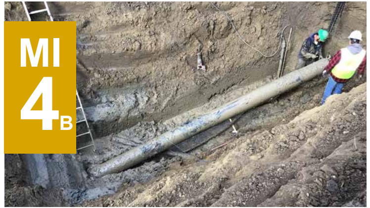
Removing the pullhead after completion of the river crossing bore.
